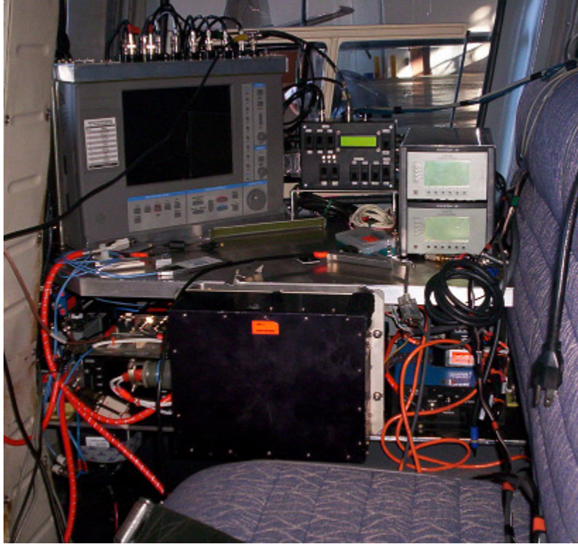
Figure 4.1: Equipment pallet installed inside Bell 206 aircraft.
