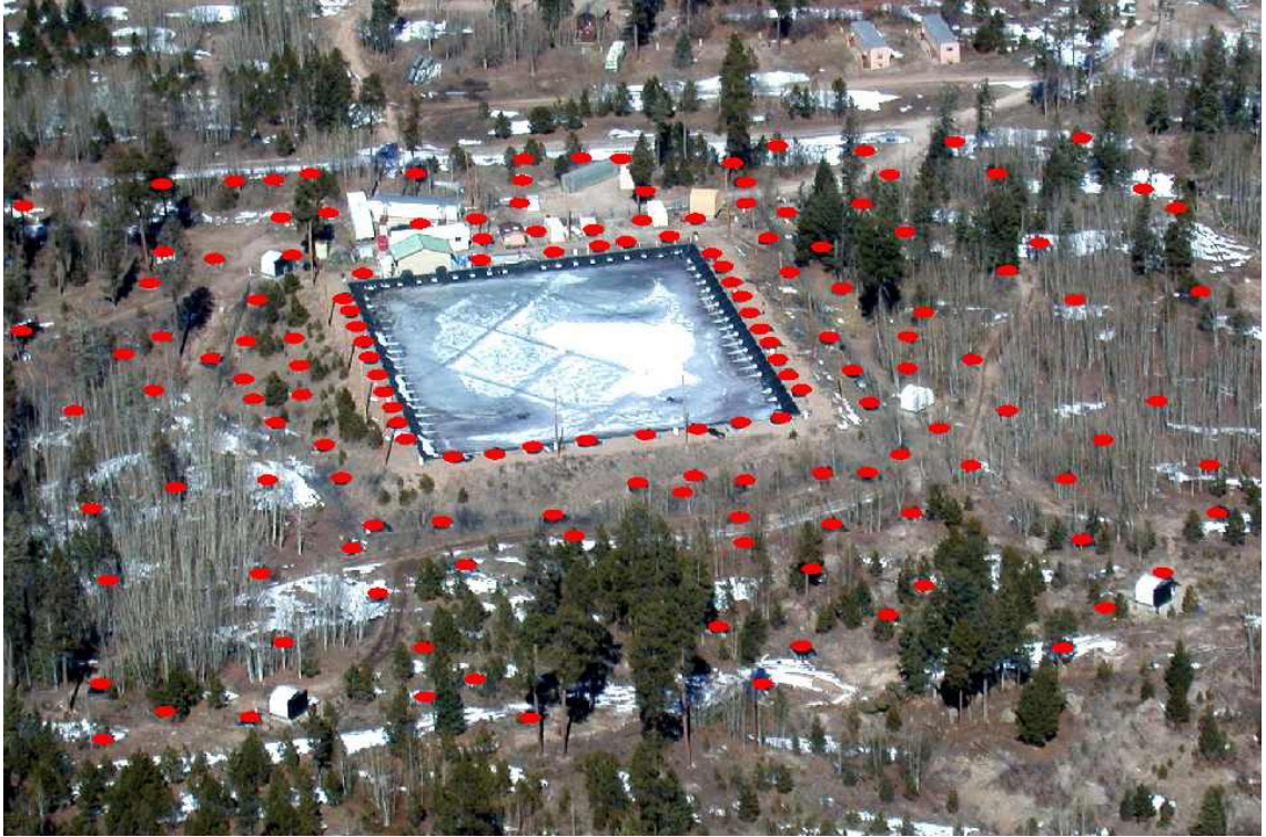
Figure 5.4: Aerial view of the complete Milagro detector. The pond, shown here with snow on the cover, is in the middle. The buildings next to the pond house the electronics, storage spaces and the water filtration systems. The outrigger array is also shown (red dots) around the pond.
