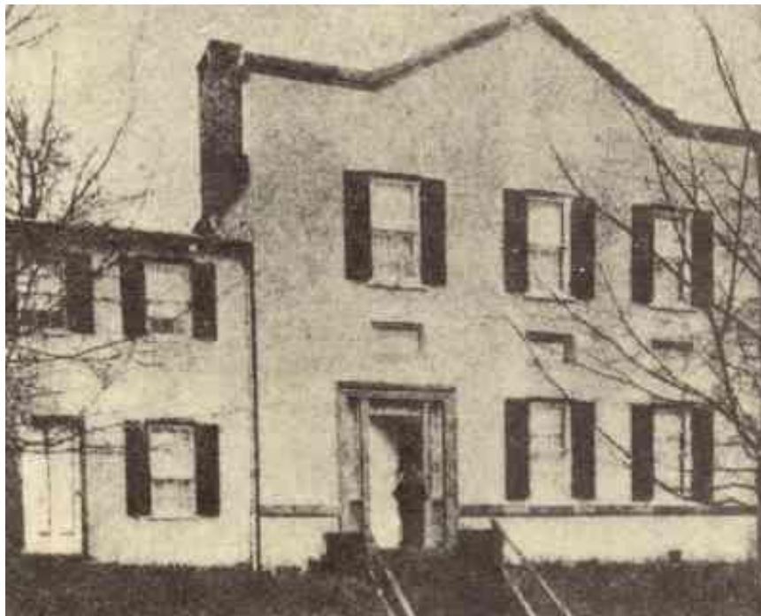
Figure 3. Old Lancasterian School This is not the actual 1811 school but of the era. (Source: DCPS Photo Gallery, www.k12.dc.us )
