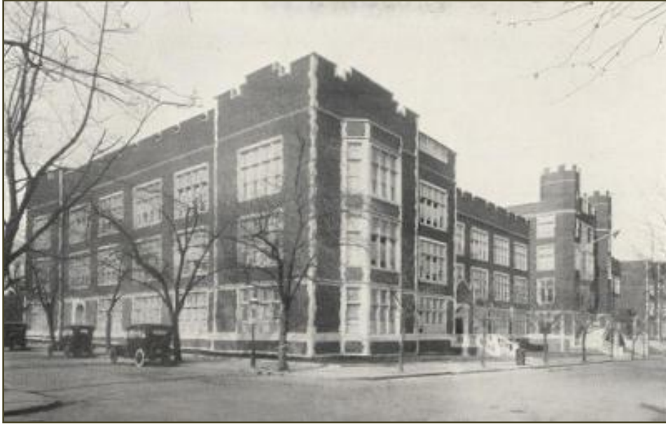
Figure 19. Old Dunbar High School, 1925. Source: DCPS Photo Gallery, www.k12.dc.us/schools.htm
