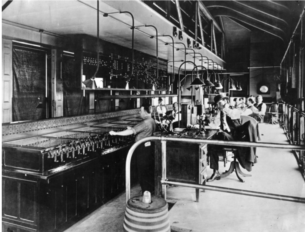
Figure 21 The “A” Tower, Pennsylvania Railroad, NYC. Maintaining these all electric interlocking systems put the BRS members in jurisdictional conflicts with the IBEW. The level and variety of their skills maintainers needed to acquire is demonstrated in the complexity of these traffic management systems. No date, File Photo, The Archives of the Brotherhood of Railroad Signalmen.
