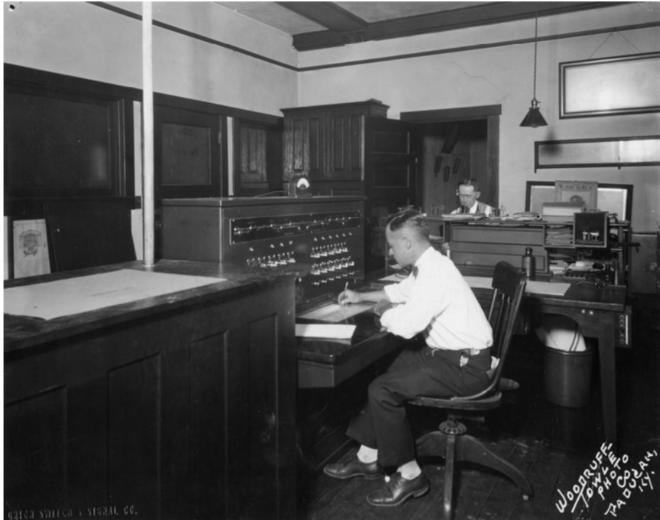
Figure 11 A Centralized Train Control office of the Paducah and Louisville Railroad, Operators could handle more traffic and larger plants with improved safety. Photo by Woodruff Towle, Paducah, KY, no date available. File photo from the Archives of the Brotherhood of Railroad Signalmen, Front Royal, VA.
