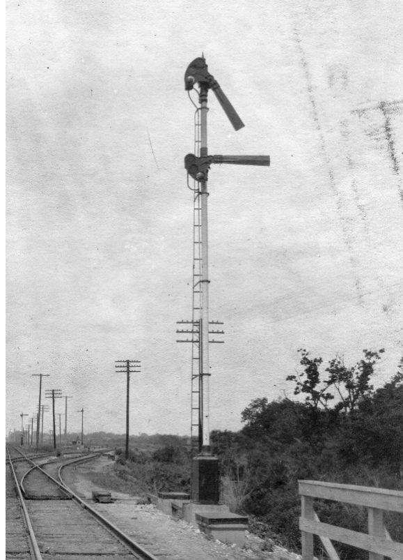
Figure 7 A set of semaphore signals, possibly giving indications for an approach to the next block or to a station block, interpretation dependent on the carrier’s instruction manual. File photo, Archive of the Brotherhood of Railroad Signalmen, no date or location.
