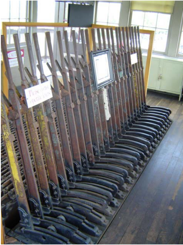
Figure 4 Mechanical Interlocking for a terminal or large train yard located on the second floor of the Interlocking Tower at the Railroad Museum of Pennsylvania, Strasberg, PA. Photo by Robert Williams, June, 2007.
