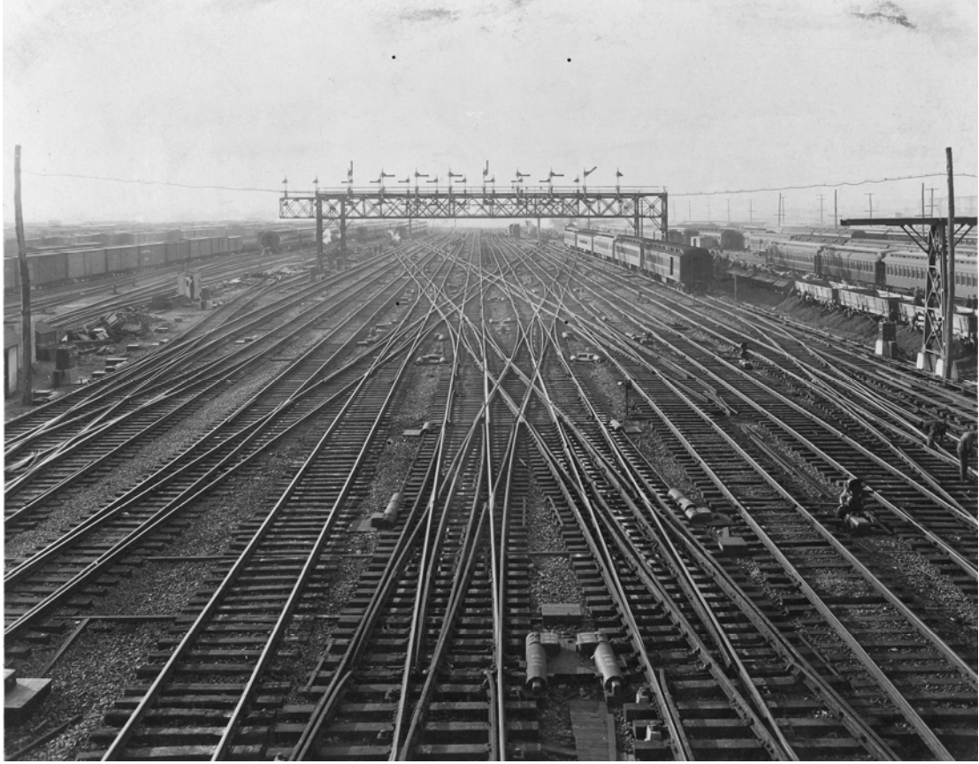
Figure 23 Signalmen installed, maintained, and repaired complicated signal systems such as this photograph depicts. File photo noted only as Signal 029, no location or date given, BRS Archives, Front Royal, VA.
