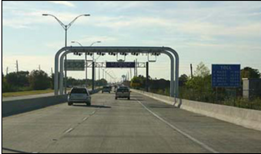
Figure 5-1: Open Road Tolling Gantry
