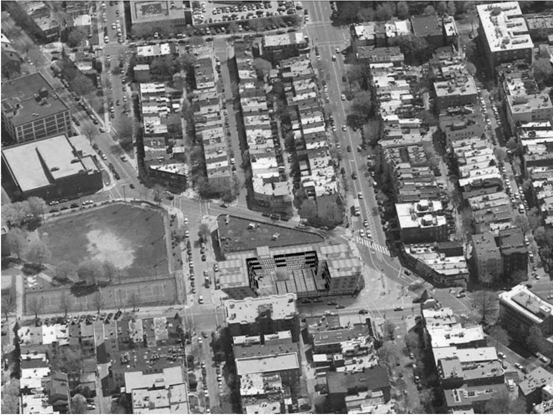
Figure 25 Aerial view of Courtyard Transitional Housing Building. North <
