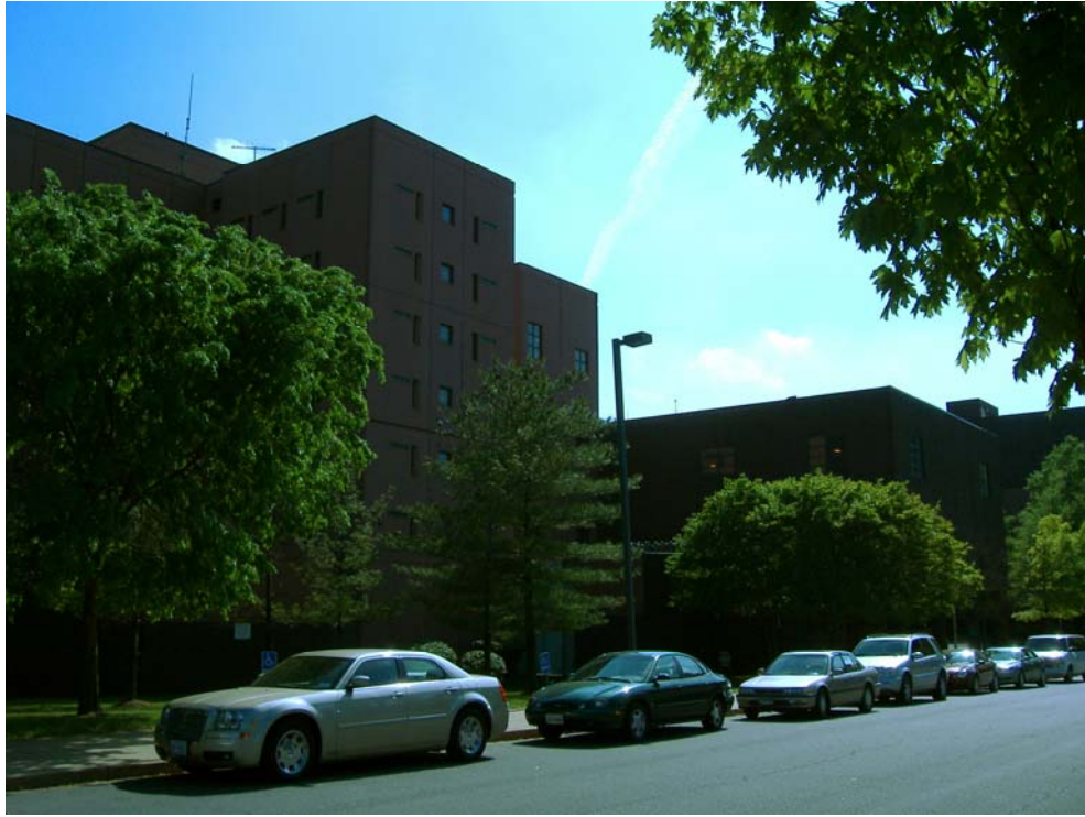
Figure 19 – Department of Corrections: Correctional Treatment Facility
