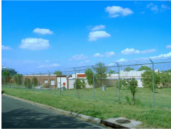
Figure 29 – DC Water and Sewer Authority (DCWASA) pump station and swirl concentrator
