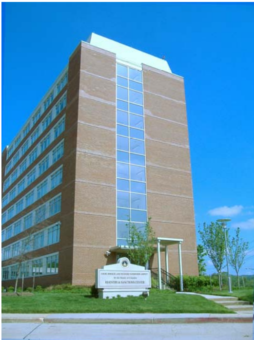
Figure 14 – Department of Health: Substance Abuse Treatment Facility
