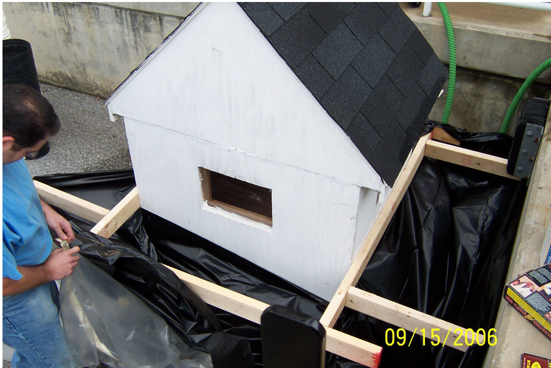
Figure 5.3. Construction of gutter system on model house.
