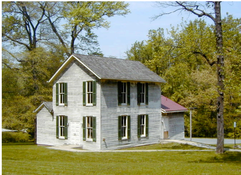
Figure 2: Abraham Hall, after restoration. Courtesy of the Prince George's County Planning Department, M-NCPPC.
