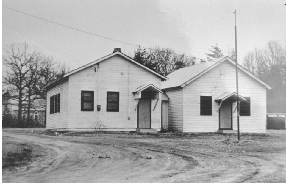
Figure 3: Chapel Hill Rosenwald School, no longer extant. 1923 building on the left, 1926 addition on the right. Courtesy of the Prince George's County Planning Department, M-NCPPC.
