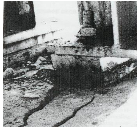
e) Frozen Bearing and Damaged Bridge Seat under Joint
