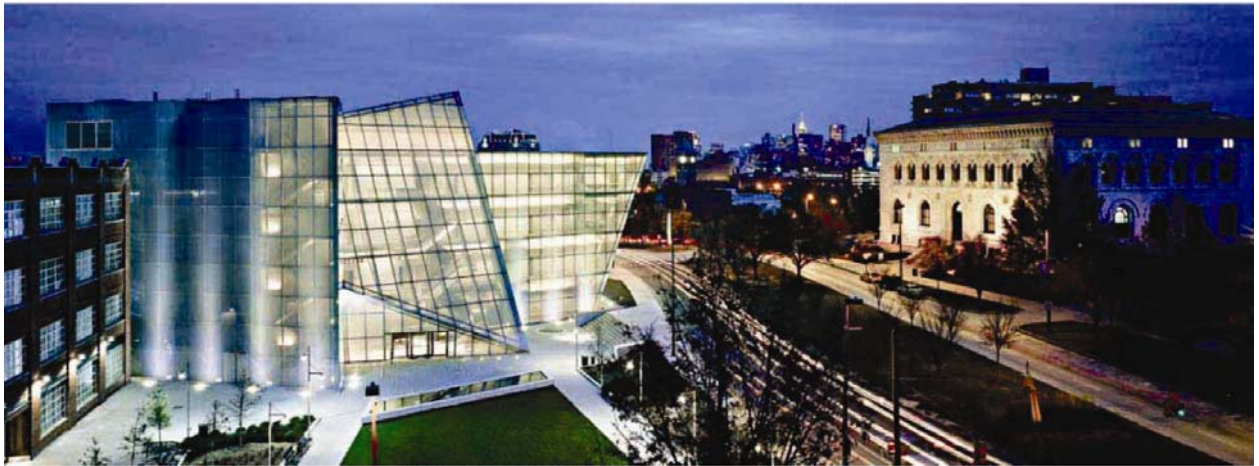
Figure 14- View of MICA Brown Center and Mount Royal Avenue.
