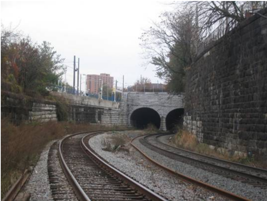
Figure 37- View of the rail line and the site's retaining wall on the right.
