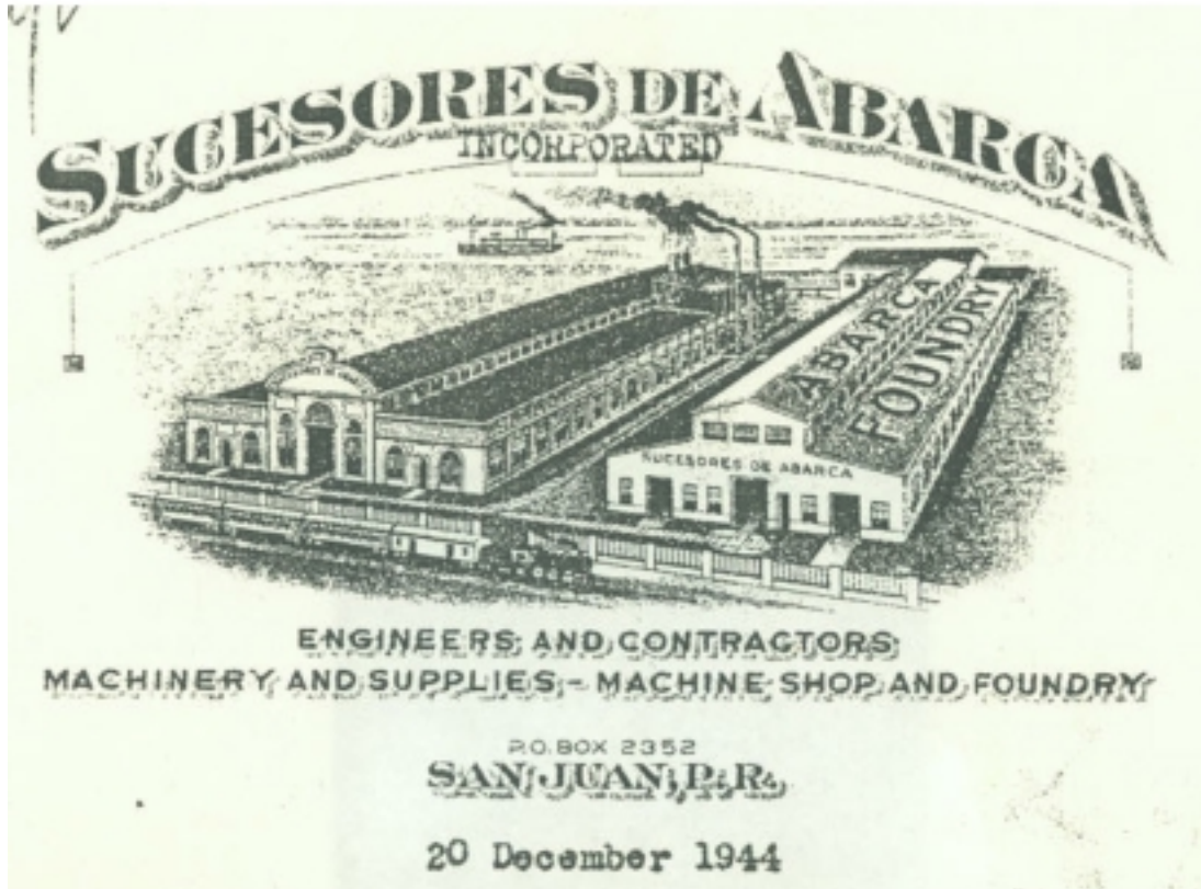
Figure 45 Aerial perspective of Fundición Abarca, 1944.
