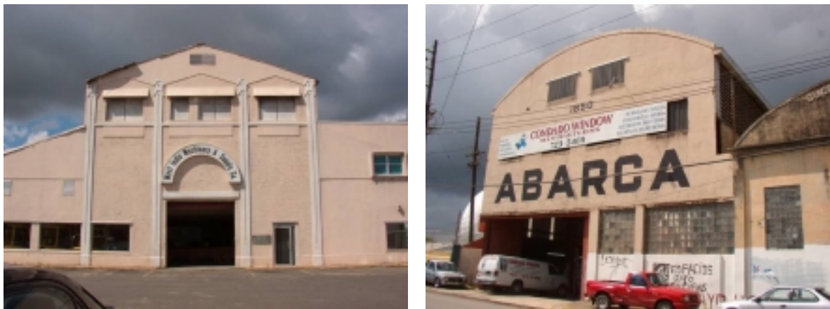
Figure 53 Fundición Abarca remaining structures B and E.
