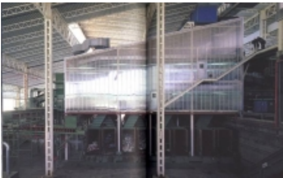
Figure 62 Madrid Recycling Plant
