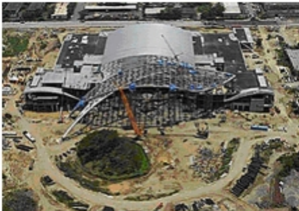
Figure 39 Puerto Rico Convention Center under construction.
