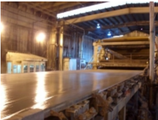
Figure 11 Flat screen drainer.
