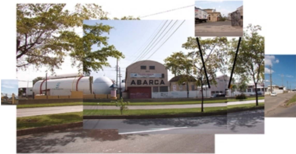
Figure 34 Existing southwest façade of Ave. Muñoz Rivera.
