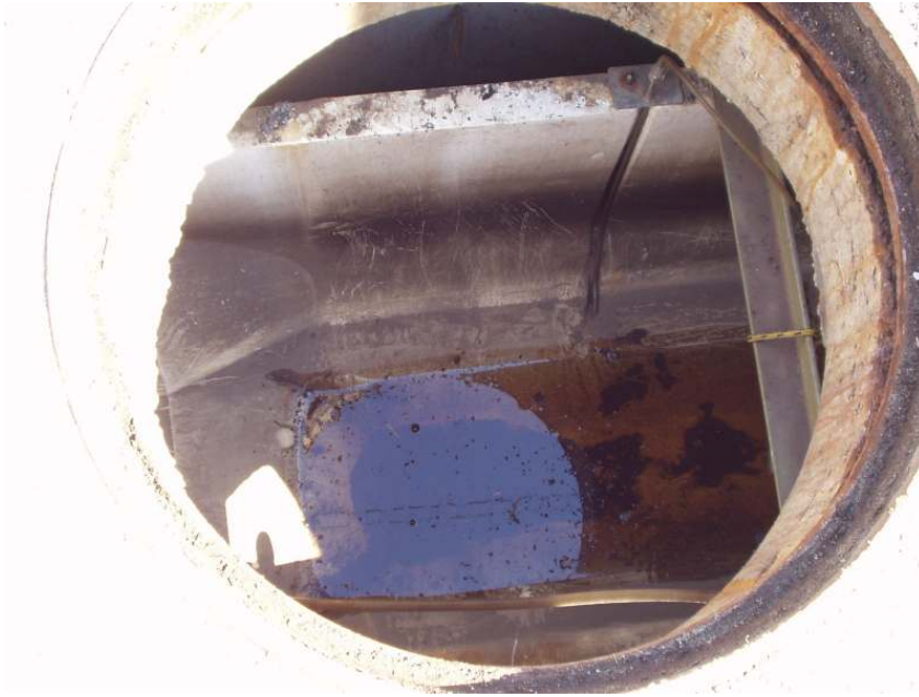
Figure 4.3. Residual water in the flume at the sampling point resulting from seepage water (March 2005).
