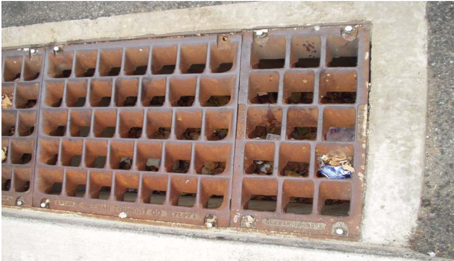
Figure 3.8. Gutter Filter on East side of Rt. 1.
