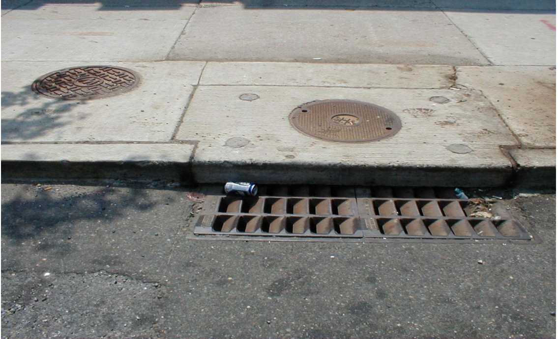
Figure A.3. East side inlet before installation of gutter filters.
