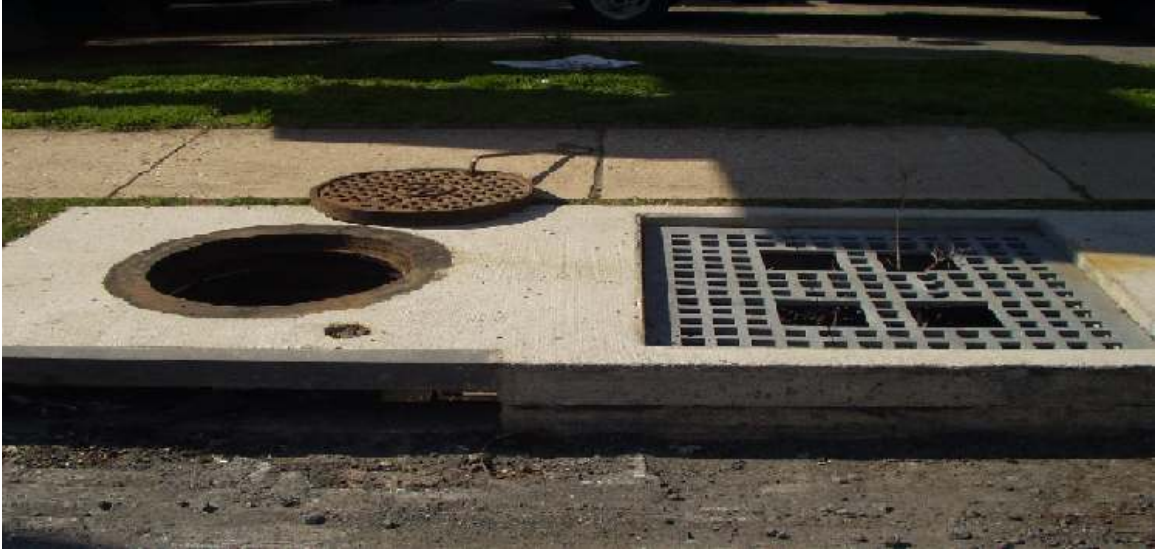
Figure 3.10. Bioinlets and the manhole for the inlet chamber (facing west) (04/2005).
