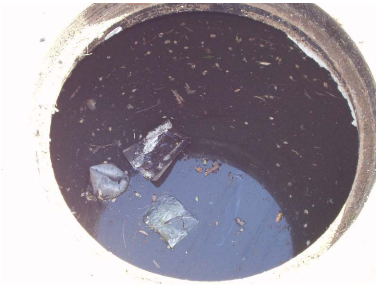
Figure 4.2. Disturbance in the pipe alignment between the inlet storage chamber and the bioinlet resulted in accumulation of water in the storage chamber (March 2005).
