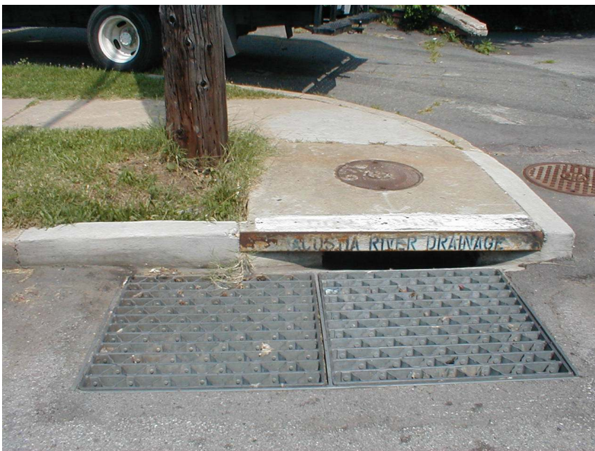
Figure A.8. West side inlet.
