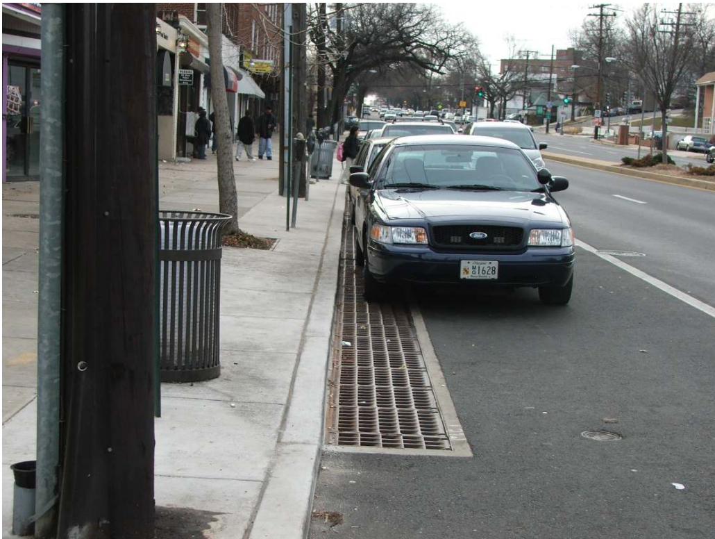
Figure A.6. Gutter Filters on the east side due south at Mt. Rainier, MD.
