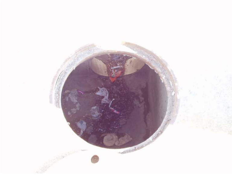
Figure 4.1. Oil residue in the flume from greasing of a nearby utility pole (March 2005).
