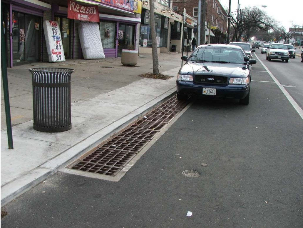
Figure A.5. Gutter filters on the east side of Rt. 1 at Mt. Rainier, MD.
