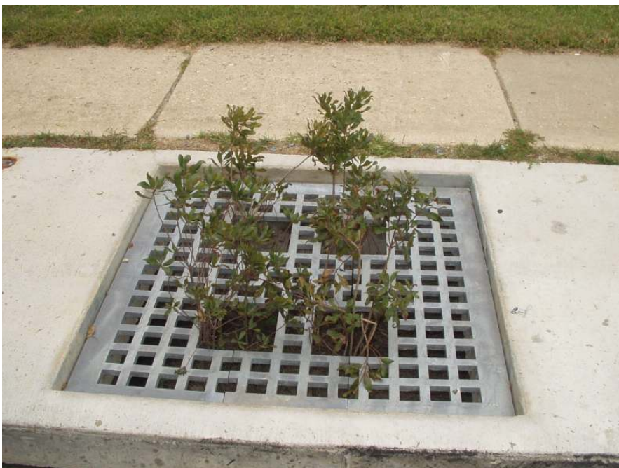
Figure 3.9. Bioinlets on the West side of Rt. 1(facing west) (10/2004).
