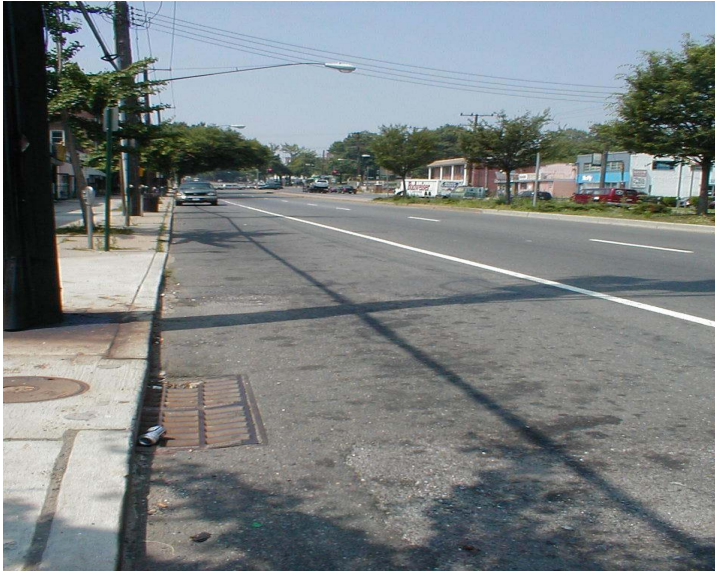
Figure 3.4. East side inlet, looking south on Rhode Island Avenue before LID.
