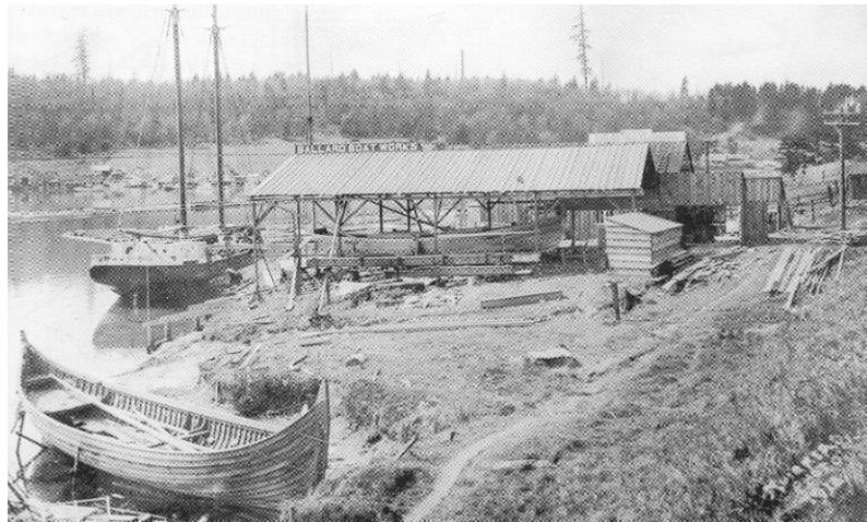
Figure 13 - Ballard Boat Works in 1905. [Passport to Ballard]
