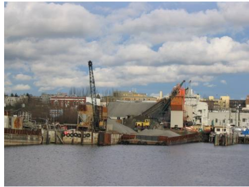
Figure 17 – (View 2) Site context: Sand and gravel yard just north and west of the site. Large barges carrying sand, gravel and cement travel up and down Salmon Bay.
