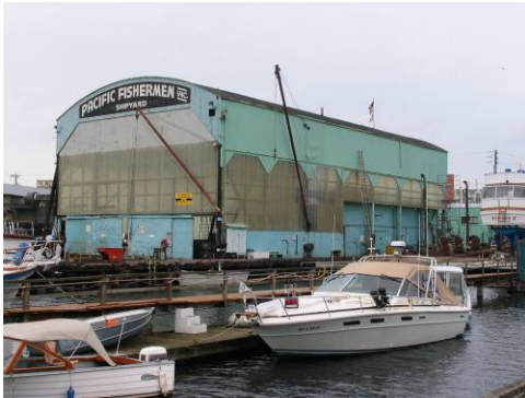
Figure 16 – (View 1) Site context: All around the site are large ship and boat repair facilities of all sizes. In addition, marina and boat storage facilities exist all along the Salmon Bay waterfront.
