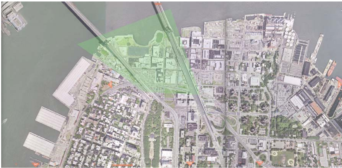
[Fig. 2] Aerial Photograph showing (from left to right) the neighborhoods of Brooklyn Heights, Downtown Brooklyn and DUMBO and The Brooklyn Navy Yard. (McGraw Hill)
