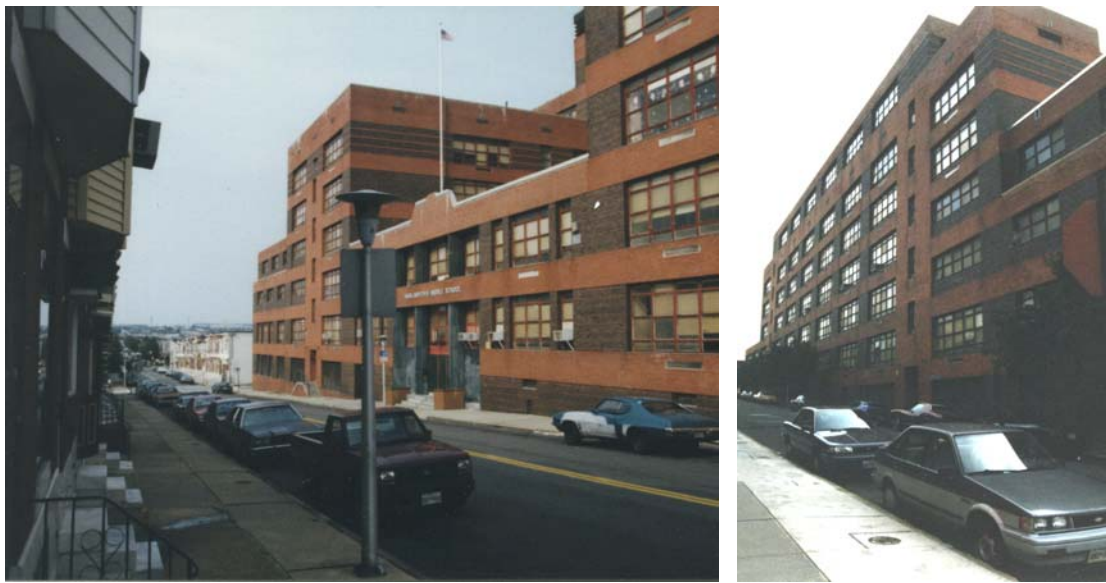
Fig. 41 & 42: Hampstead Hill Middle School On the west side, the school is two stories high at the center, respectful of the residential scale. On the east side the building towers over the street.
