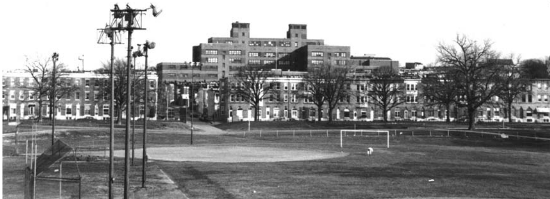
Fig. 43: Hampstead Hill Middle School The view from Patterson Park - The school towers over the neighborhood.
