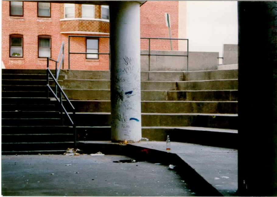
Fig. 35: Space Beneath Highlandtown Elementary School A space designed for children, the space beneath Highlandtown elementary school, with its accumulation of litter, graffiti, and beer bottle, represents the least maintained area in the entire neighborhood.
