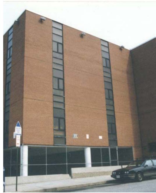
Fig. 32: Facade - Highlandtown Public Elementary School
