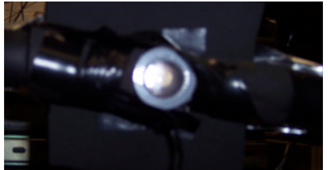
Figure 33 – Gas Line Sight Glass with Moisture Indicator
