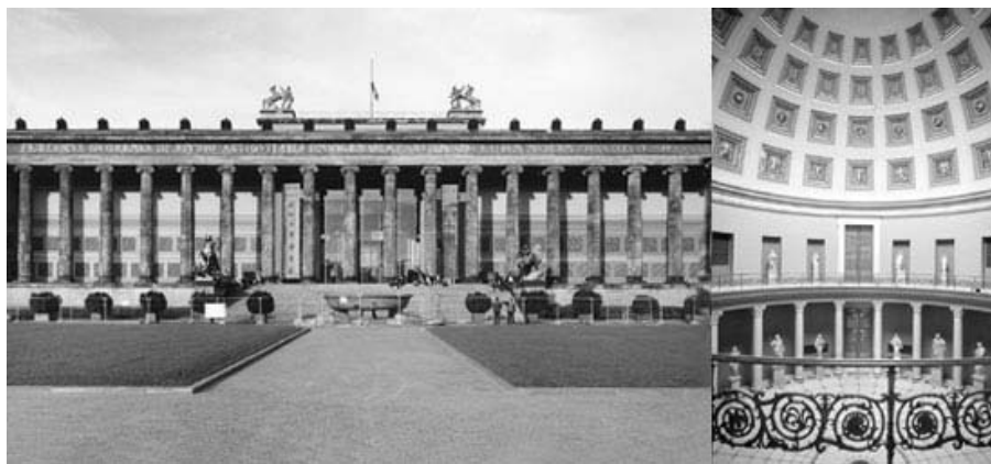
Figure 3: Altes Museum by Karl Friedrich Schinkel. View showing the colonnaded portico and the "sanctuary," the rotunda which organizes the building.
