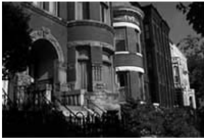
Figure 9 : Streetscape in Capitol Hill that is typical of what residential Washington DC looked like in the late nineteenth century.
