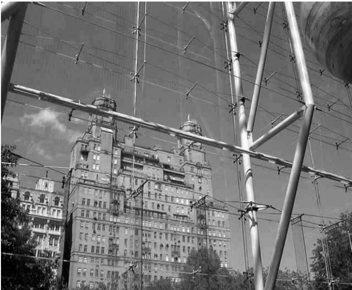
Figure 43: This view from within the Rose Center shows how the transparent walls allow the historic architecture surrounding the site is allowed to be the backdrop for the experience in the building.
