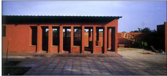
Fig. 75: Open structures allow for cross ventilation
