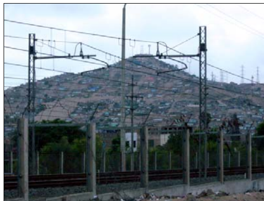
Figure 16: Electric train right of way along Industrial Separator Ave.
