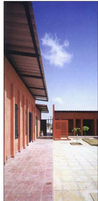
Fig. 76: View of exterior circulation. Wide eaves provide protection against the sun.
