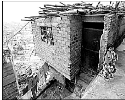
Photo: Precariously built home in El Pino, northern district of Lima.
