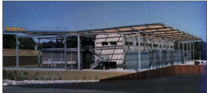
Fig. 82: Exterior view showing the outdoor spaces created by the canopy. It also shows the duality between solid heavy construction and light and airy design.
