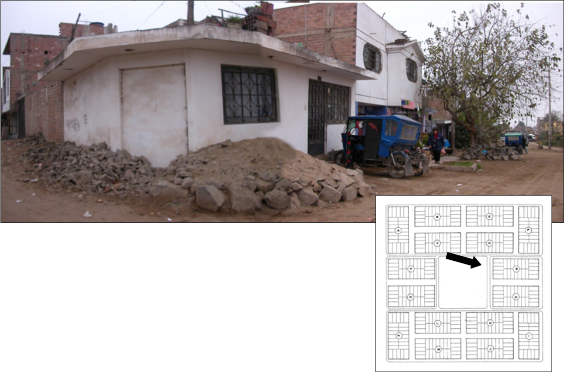
Fig. 53: Facades Side A1
