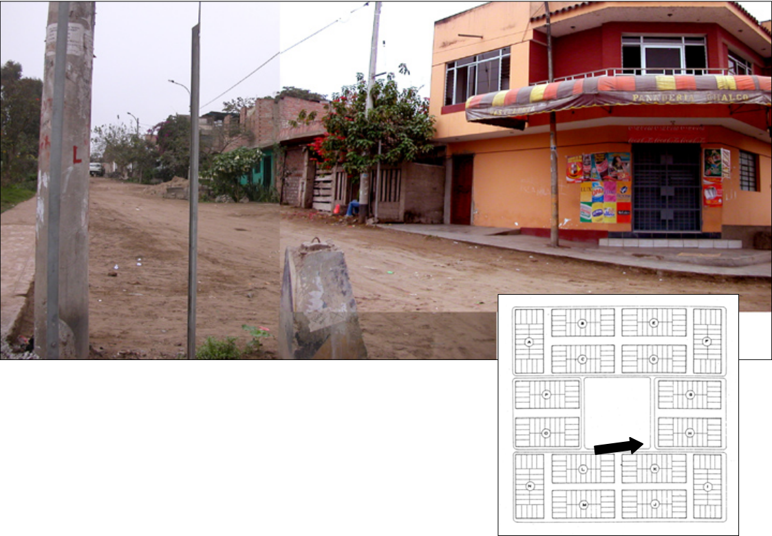
Fig. 54: Facades Side A2
