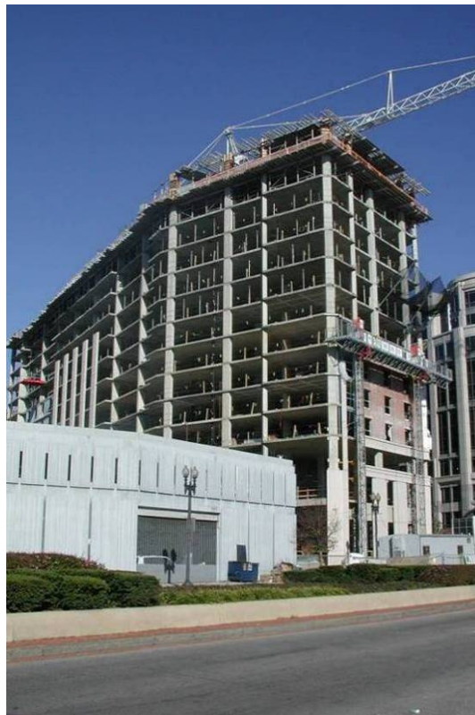
Figure 55-Image showing the new 15 story hotel currently under construction
