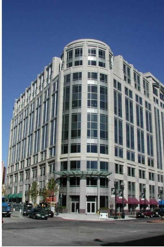
Figure 56-Image showing the new 12 story office building to the north of the site
