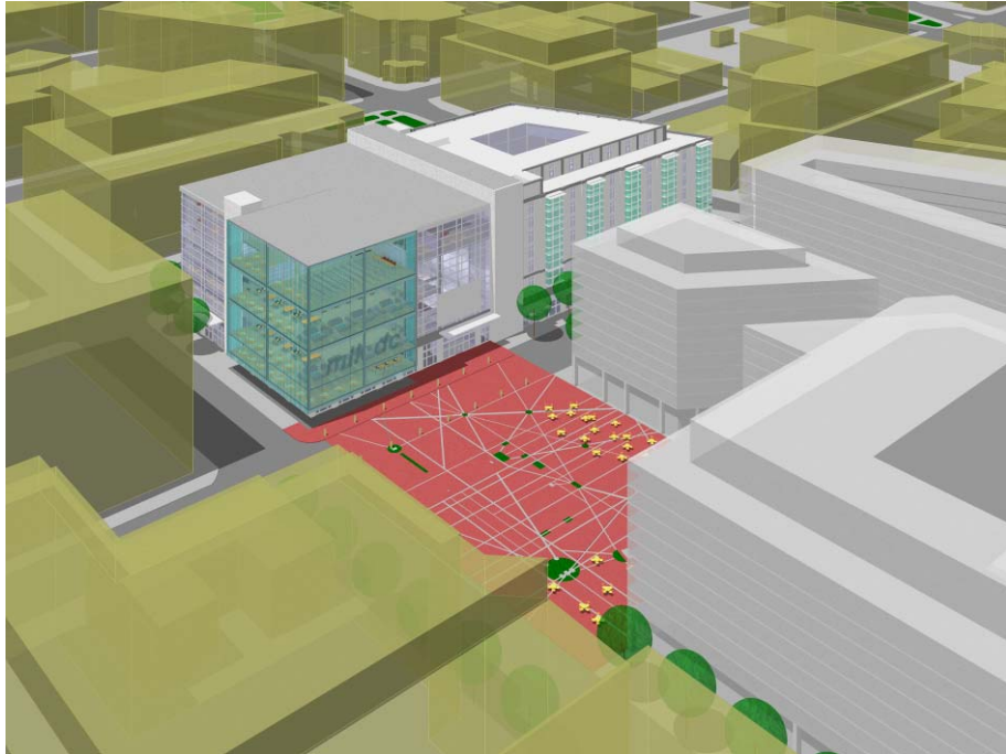
Figure 121-Aerial view showing the three main elevational parts of the library, the translucent prism, the clear glass curtain wall, and the opaque buffer between the library and the mixed-use building to the north
