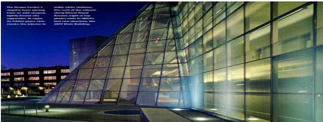
Figure 90-Picture showing relationship between the Brown Center, and the existing Fox Building (Architectural Record)
