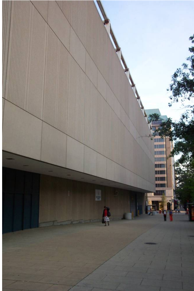
Figure 15-Image showing detailing of the western wall, and its relationship to 11th street
