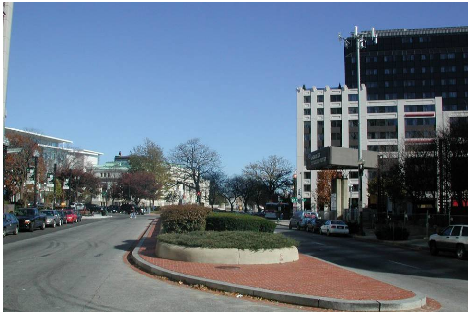
Figure 57-Image showing the character of New York Avenue to the north of the site-and the relationship of the 14 story office building, the new convention center, and the Carnegie Library
