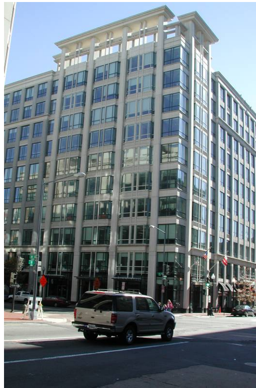
Figure 47-Image showing the 10 story office building to the southeast
