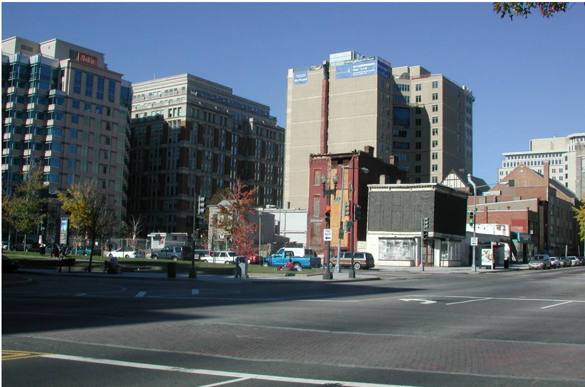
Figure 53-Image showing the 2-3 story abandoned retail buildings to the northwest of the site
