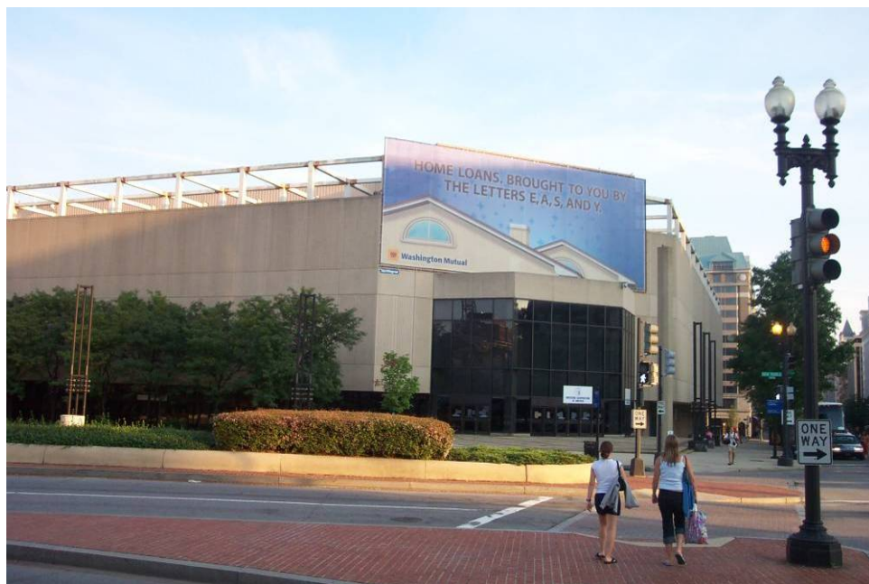
Figure 12-Image from the northwest corner of the building, from New York Avenue and 11th street
