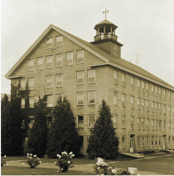
Figure 10. Enfield Shaker Village Dwelling. Historic American Buildings Survey, The Library of Congress.
