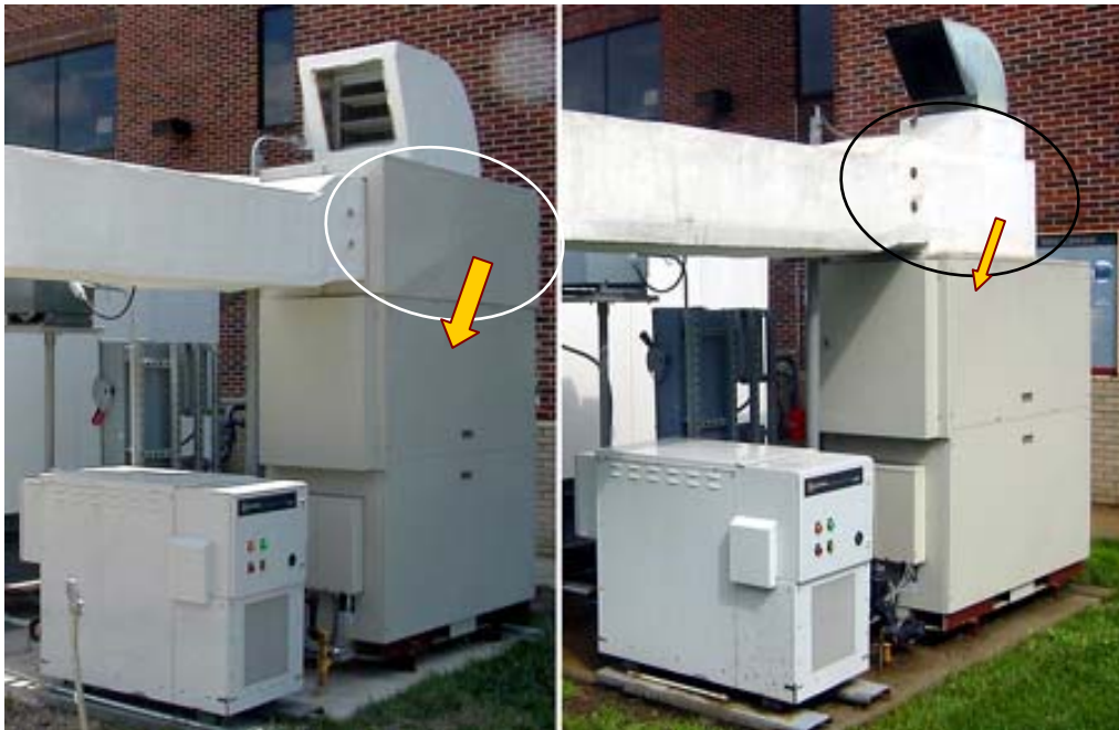
Fig. 82. Two kinds of plenum box (with circle) installed on the top of MT
