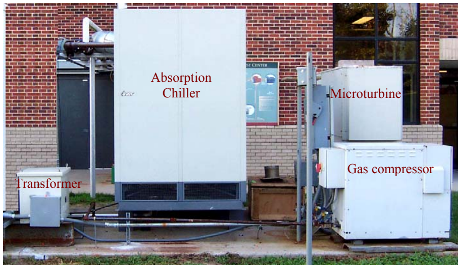
Fig. 80. The simplified third-generation MT-based system
