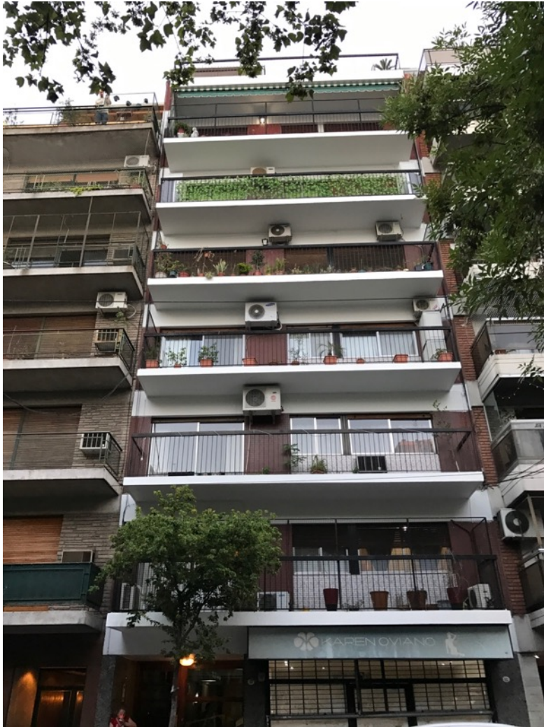
Figure 45: Balconies are often Personalized (Author)
