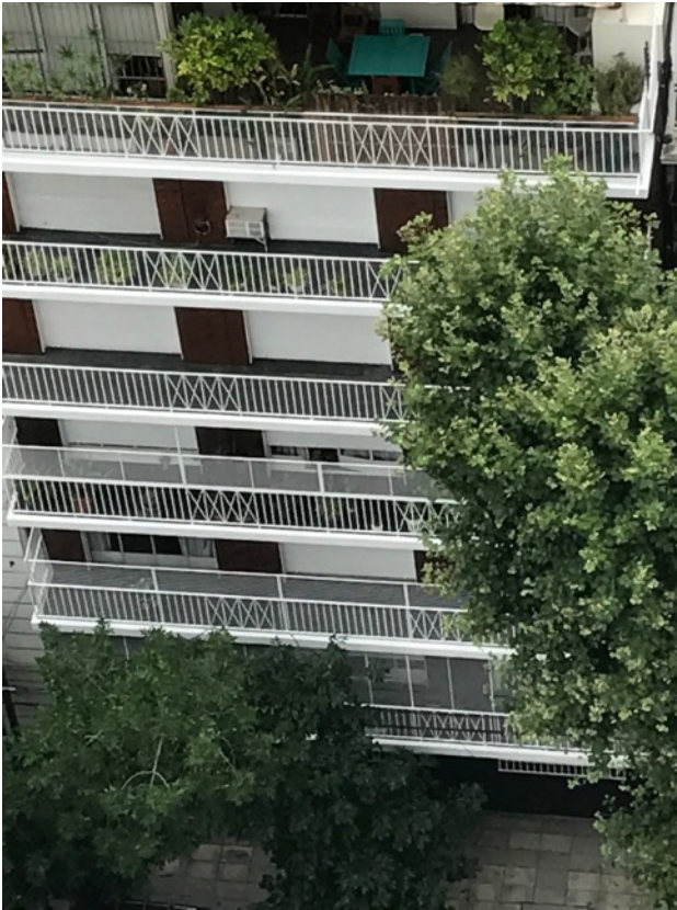
Figure 46: Apartments Shut Out Sun and Light from Inside Spaces (Author)
