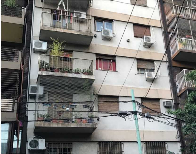
Figure 19: Air Conditioning Units on Facade (Author)
