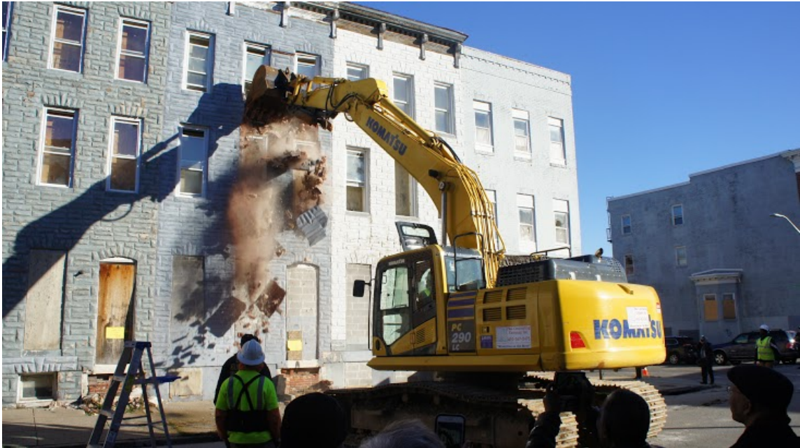
Figure 4. Project C.O.R.E. demolition in Sandtown-Winchester (Department of Housing and Community Development, 2016).
