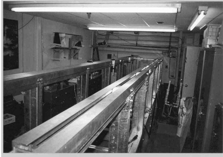
Figure 4.4: Aluminium L-beams mountings for the carriage rails during the construction process
