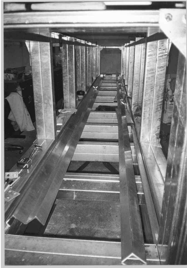
Figure 4.1: Tank structure during the alignment process.
