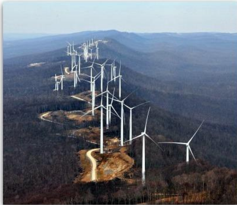
Figure 6-22 Installed Turbines on the ridge of the mountain
