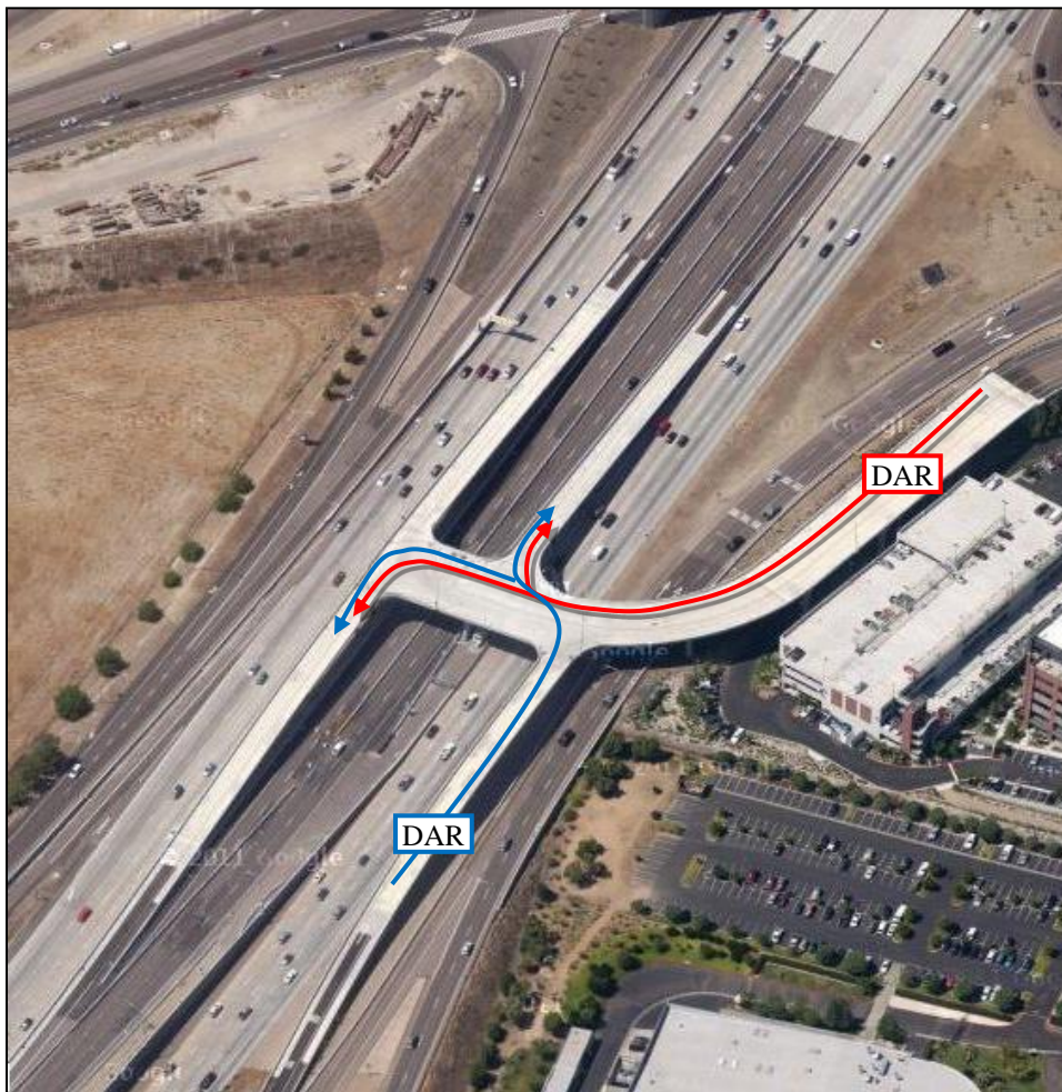
Figure 43. Direct access ramp (DAR) for entering (and exiting) the I-15 Express Lanes, California (Source: Google Maps 2011).
