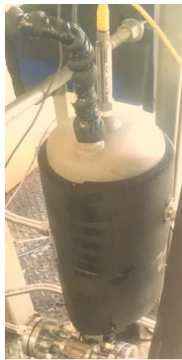
Figure 29: Ammonia Liquid Receiver
