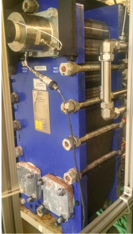
Figure 28: Alfa-Laval M10BW-FD PHE Condenser
