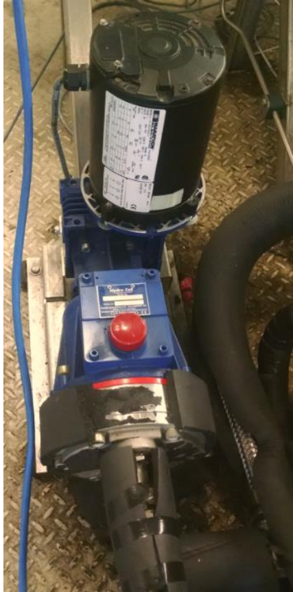
Figure 26: Ammonia Pump with VFD Motor
