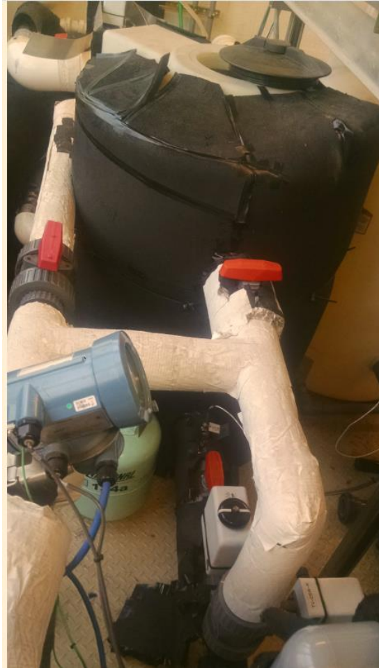
Figure 19: Cold Water Tank and Coriolis Flow Meter
