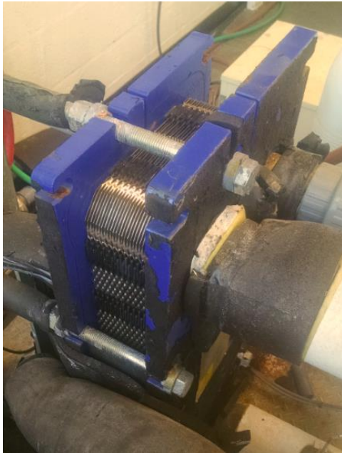
Figure 21: Water-Glycol Heat Exchanger
