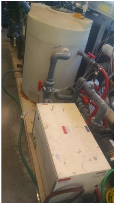
Figure 17: Warm Water Tank with Electric Heater
