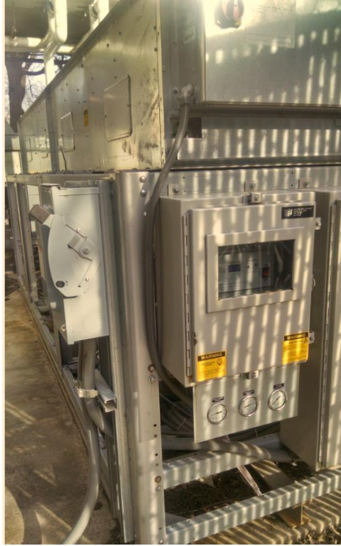
Figure 20: Outdoor Glycol Chiller
