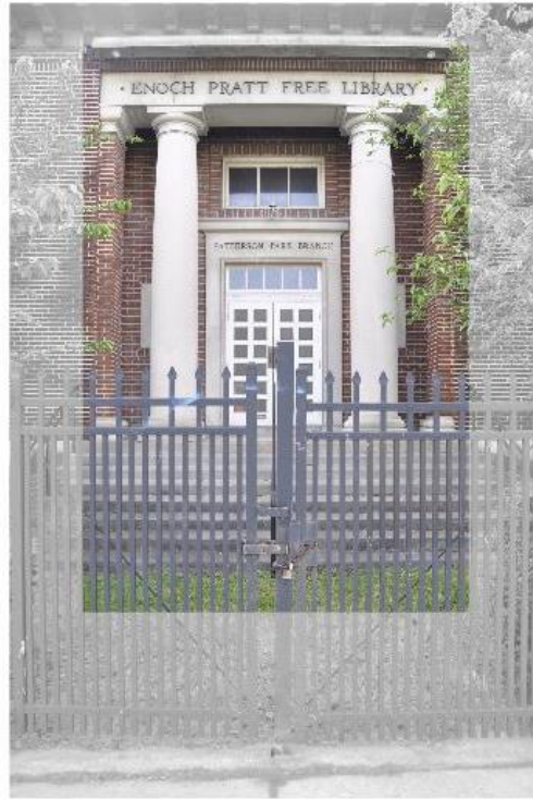
Figure 19 Entry Facade (Image by Author)
