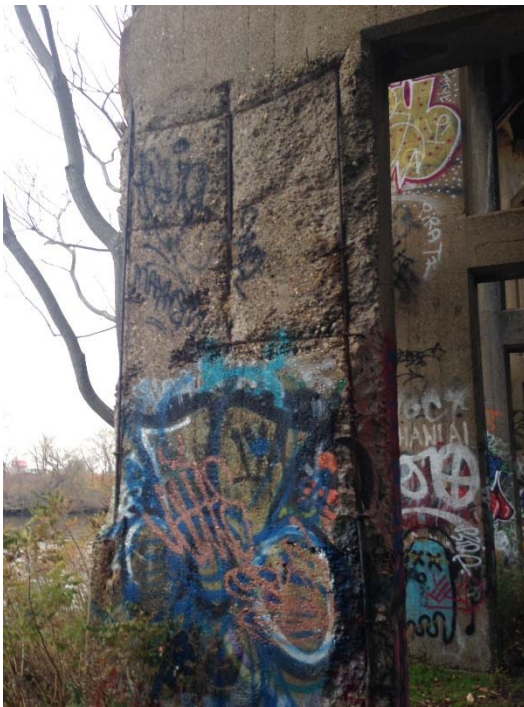
Figure 27: Pier 124 exposed rebar, source: Author
