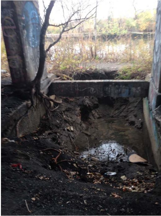
Figure 29: Pier 124 vegetation penetrating structural grid, source: Author
