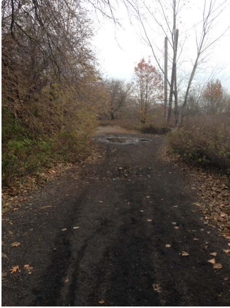
Figure 32: Pier 124 Approach from Beach St., source: Author
