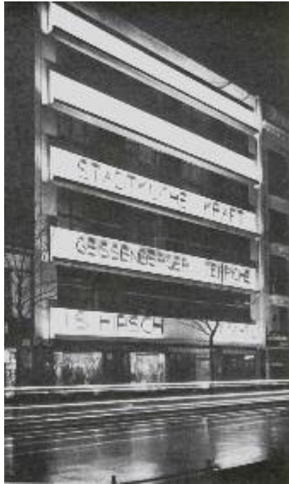
Fig. 23 Wassili and Hans Luckhardt and Alfons Anker. Office Building, Berlin, 1925. Reproduced in Arthur Korn, Glass in Modern Architecture of the Bauhaus Period.
