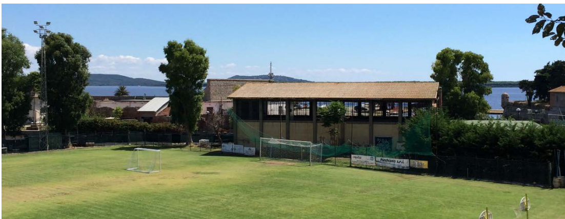
Figure 35: View of Warehouse from the Wall, Credit: Author
