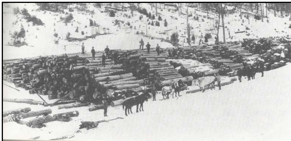
Figure 3: A skidway of logs located near the Allegheny River. 16
