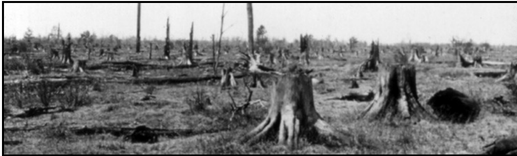
Figure 4: Stumps left behind after removing timber. 21
