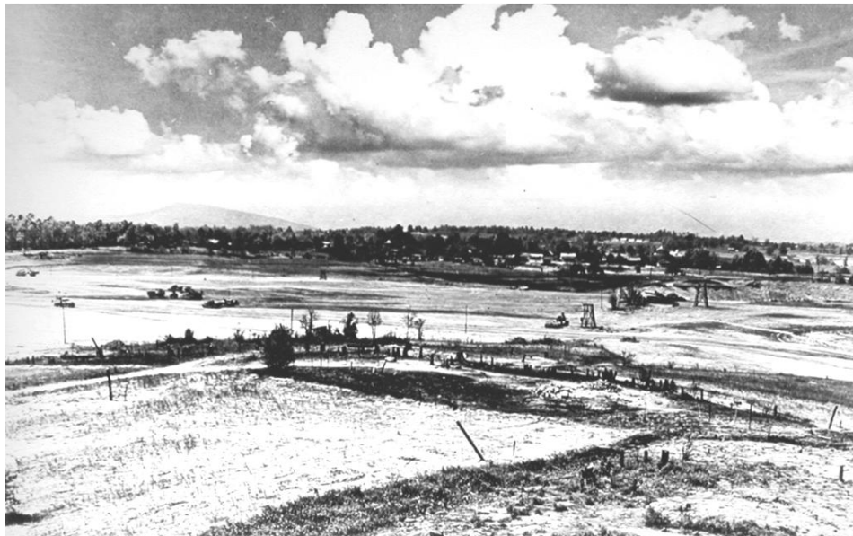
FIGURE 18: SITE OF FUTURE BELL BOMBER PLANT, c. 1942 Photograph Collections, Marietta Museum of History, Marietta, Georgia, D3.17.5.
