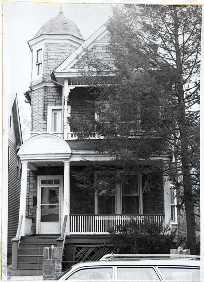
Figure 5-2 Typical Brookland Residences, c.1900
