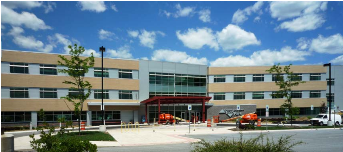
Figure 16: Greater Johnstown Technology Park. http://www.lrkimball.com/Federal_Architecture_Facility_Design_and_DB.aspx
