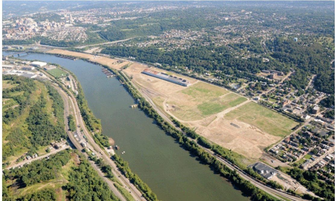
Figure 28: Aerial of the Almono Steel mill site. http://www.popcitymedia.com/features/development102214.aspx
