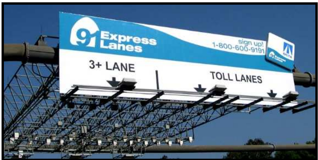
Figure 6: 91 Express Lanes Gantry & Sign
