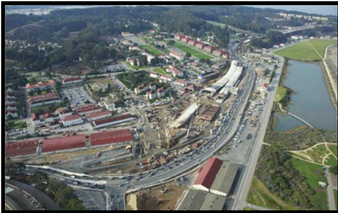
Figure 7: 2014 Aerial View of the Presidio Parkway in construction
