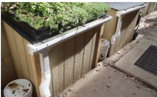
Figure 81 Accessible Green Roof
