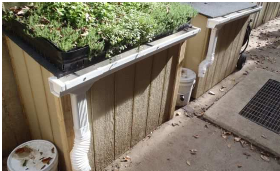
Figure 47 Brent Elementary Green Roofs
