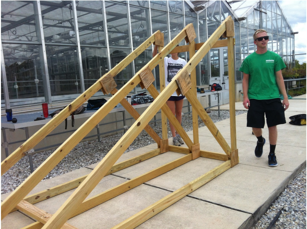
Figure 32. Truss frame of 30 degree module taken in Sep. 2012 (Courtesy of Ben Borchers)
