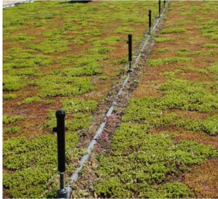
Figure 31. Overhead Irrigation System (Green Roof Tech 2013)
