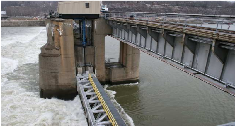
Figure 57: Spillway gates at Little Long
