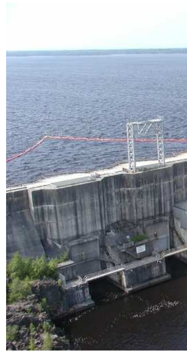
Figure 13: Little Long Generating Stations
