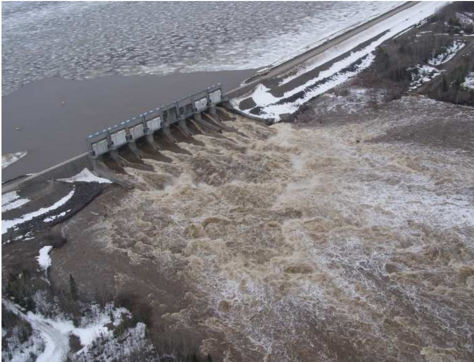
Figure 12: Little Long GS Adam Creek Spillway Gates
