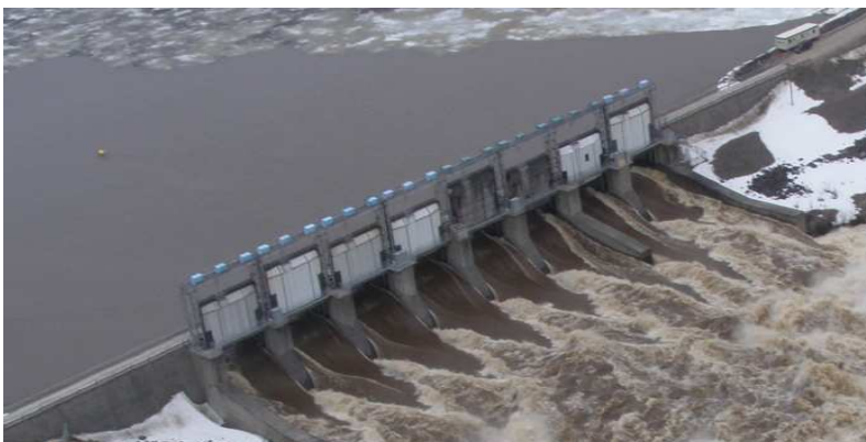
Figure 56: Spillway gates at Little Long
