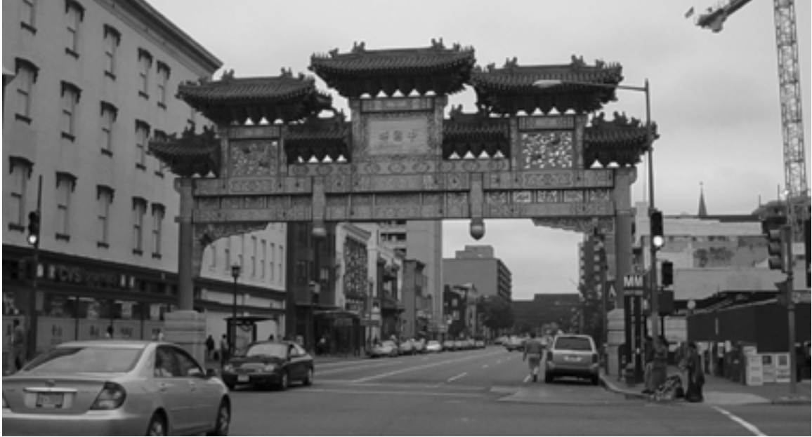
Figure 14: The Chinatown Friendship Arch. Completed in 1986, the arch acts as the focal point of Chinatown. The arch is a testament to the coexistence of Chinese and American culture combining Chinese dou gong carved wood roofing with steel and reinforced concrete support.
