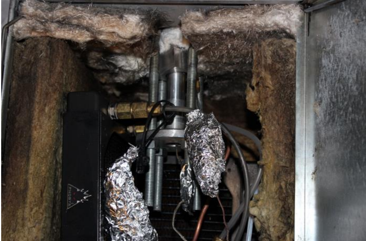
Figure 4-15 Box Interior with Instrumentation
