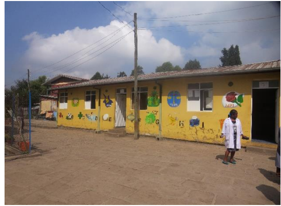
Picture of the School 2: The school compound.
