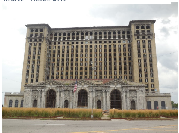
Figure 23 Michigan Central Station primary elevation. Source – Author 2013
