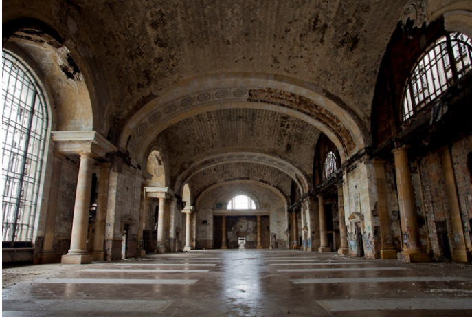
Figure 20 Image of the Guastavino Vaulted waiting room of Michigan Central (Source - Detroit Free Press 2013)
