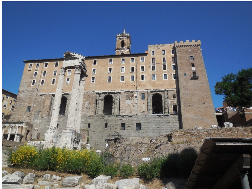
Figure 31 Palazzo Senatorio on Capitoline Hill in Rome, looking from the ruins of the Roman Forum. Remnants of Ancient Roman, Medieval and Renaissance interventions are visible here accounting for 2000 years of history. The building is still in use today as the meeting place for Roman legislators. Image by - Author 2013
