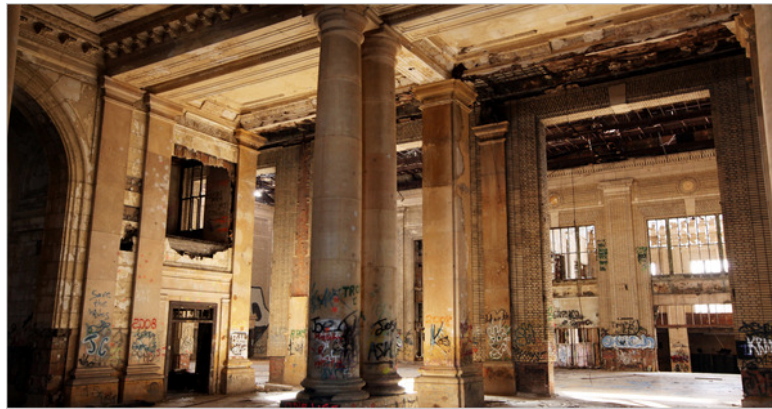
Figure 19 Image from the ticket lobby looking toward the main concourse (Source - Detroit Free Press 2013)
