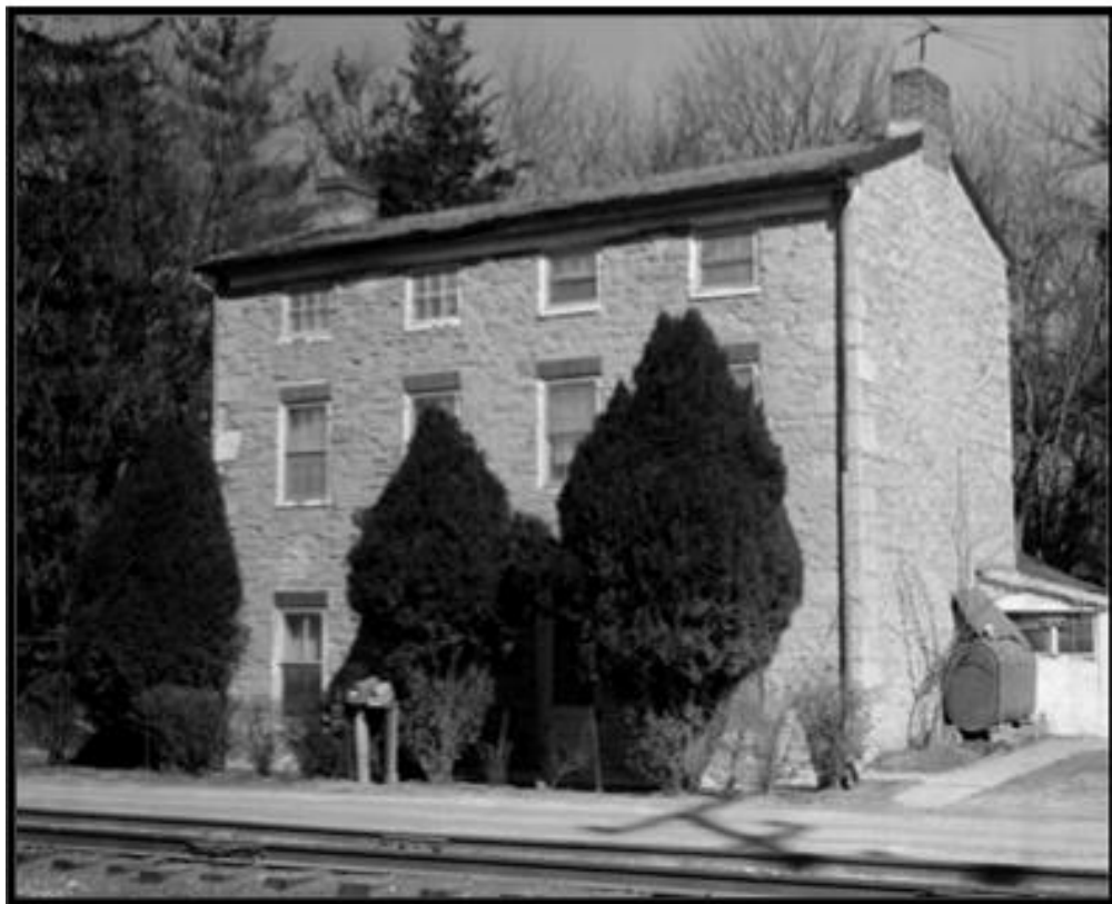
Figure 6.1: Poe-Burns Duplex. (Photographed by Herbert Harwood, Jr. 1987, photo courtesy of the Baltimore County Public Library photograph collection).
