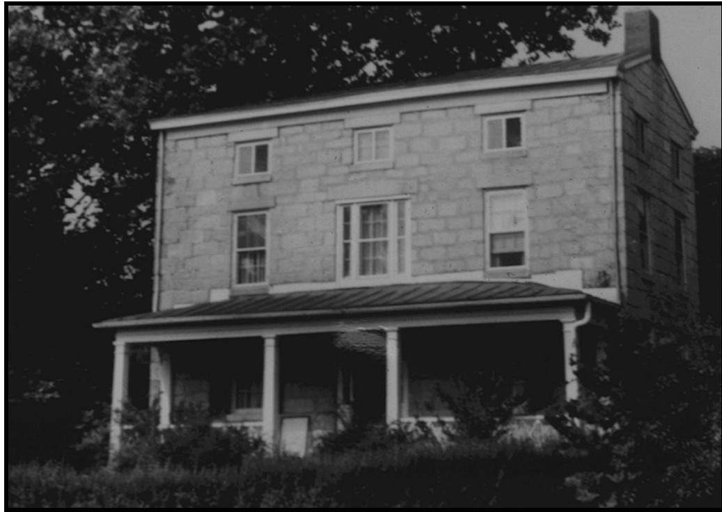
Figure 6.2: Thomas Fortune House. (Photographed by John McGrain, photo courtesy of the Baltimore County Department of Planning).
