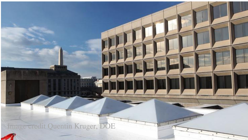
Figure 1: Example of a cool roof on a government building in Washington D.C.
