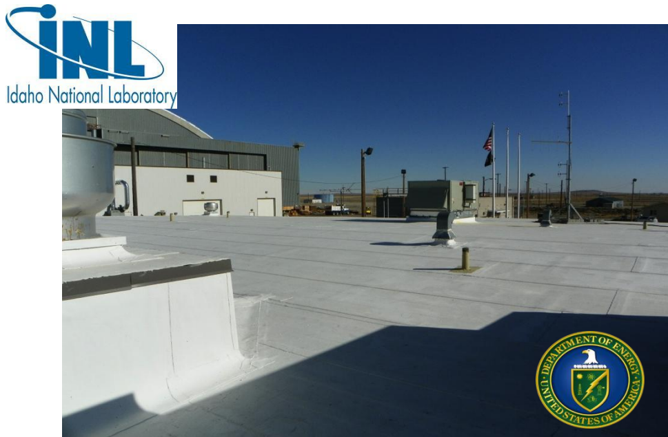
Figure 5: Idaho National Laboratory (INL) cool roof
