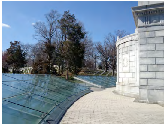
Figure 38 View of the skylights into the underground space
