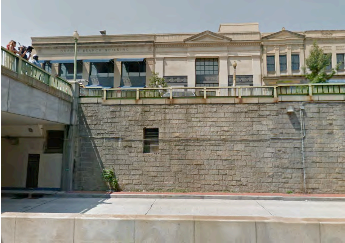
Figure 28 Poorly cut ventilation outlet in the granite wall of the Connecticut Avenue underpass, Google street view.
