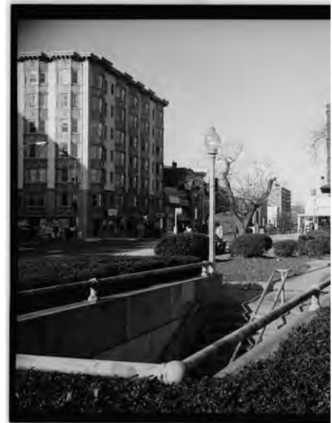
Figure 10 Reservation No. 59, Looking West with Entrance to Underground Streetcar Platform in Foreground, 5x7
