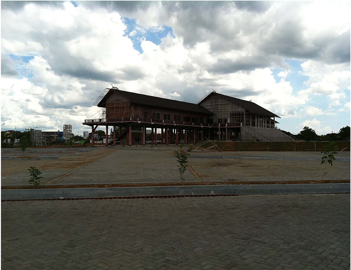
Figure 7.4: New Dayak Longhouse Under Construction in Pontianak, 2013
