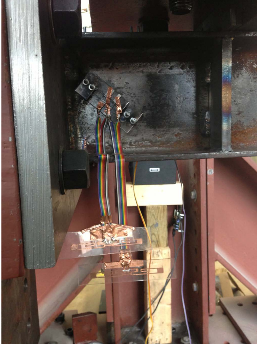
Figure 7- 22. Close-up view of BT strain sensor installed on shear link web
