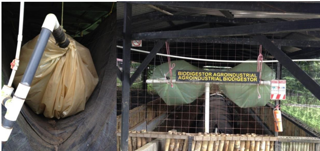
Figure 4-1. Un-mechanized, anaerobic digesters treating agricultural waste on the campus of EARTH University (Limon, Costa Rica). Photo on left shows biogas collection in polyethylene bags with PVC connections. Photo on right shows a two-stage digester treating swine waste, along with suspended biogas collection bags.
